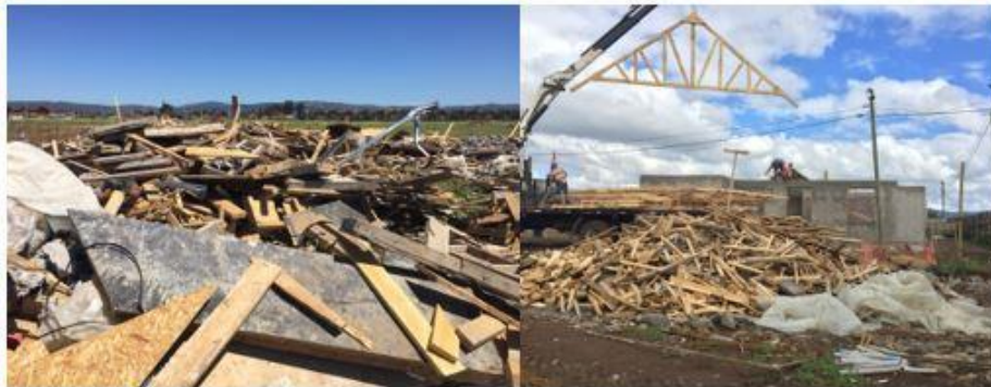
Figure 1. Construction waste in the work studied.
